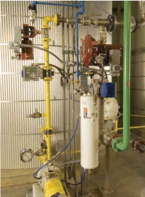
intelligence; and a choice of versions. Finally, our Coriolis mass flowmeters provide breakthrough measurement of even entrained air flows.
