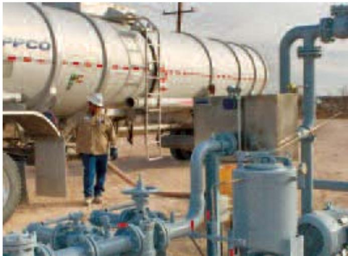
LACT units are designed for automatic transfer of ownership between buyer and seller. Here, a Foxboro CFT50 is used for truck unloading of crude with LACT unit.
