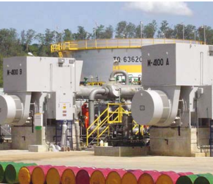
Synchronous Motors SEF900 (Ex-p), 3600 kW, 13,200 V. Application: Reciprocating compressors.
